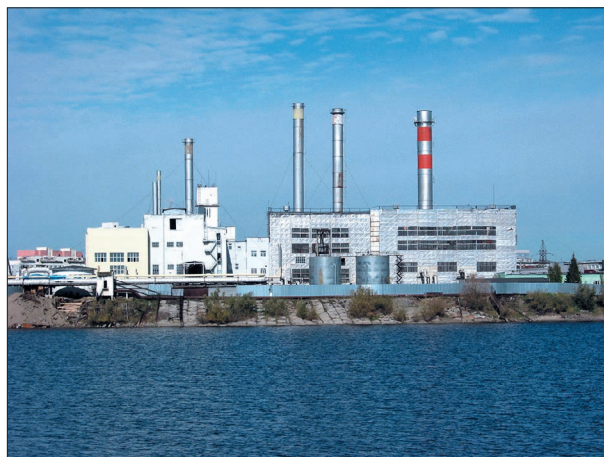
Fig. 2. A general view of the Yakutsk Combined Heat and Power Plant. (A photo by P.S. Zabolotnik, 05.09.2013).
