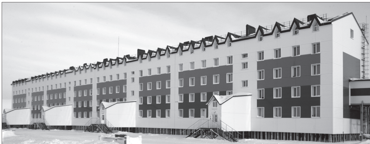
Fig. 2. The building of the dormitory on reinforced concrete piles in continuous permafrost zone, Kharasavey settlement, the Yamal Peninsula.
