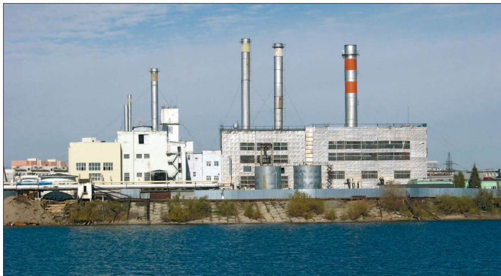
Fig. 1. A general view of the Yakutsk CHPP.
