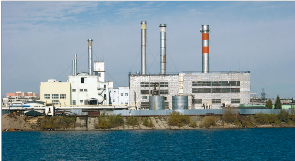
Fig. 1. A general view of the Yakutsk CHPP.
