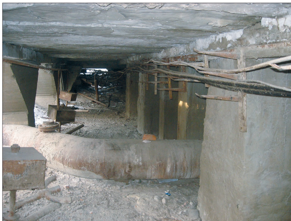
Fig. 6. The cross ventilated basement under the main building of the Yakutsk CHPP.
