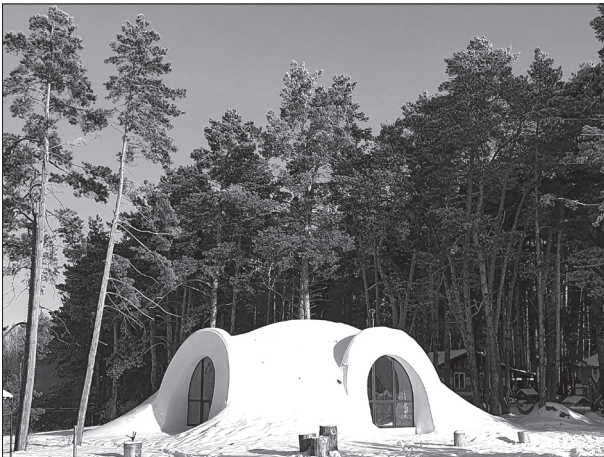
Fig. 5. Dome-shaped building made of granulated foam glass ceramics.
