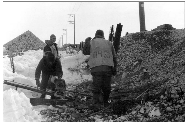
Fig. 17. Drilling of an inclined borehole (by a UKB-12.5/25 drill).
